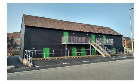
The building was constructed with strip foundations and concrete pads with a ground bearing concrete slab. The superstructure is steel frame with timber stud infill, precast plank first floor and a timber rafter roof.
