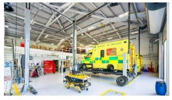
foundations, structural steel frame, hybrid in design, with a portal to the Make Ready and Fleet areas; steel roof deck with warm roof detail to the three-storey office area and a composite Kingspan roof system to the MRC/Fleet areas.
