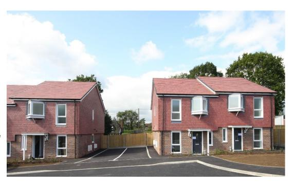
Work commenced with the installation of CFA piled foundations, with ground beams and beam and block floors. The superstructure is traditional masonry, cavity walls with block and face brickwork. The first floors are constructed using JJI joists with CaberDek flooring. From the first floor to the roof, the cavity walls are tile hung with roof trusses clad with interlocking Old English concrete tiles.
