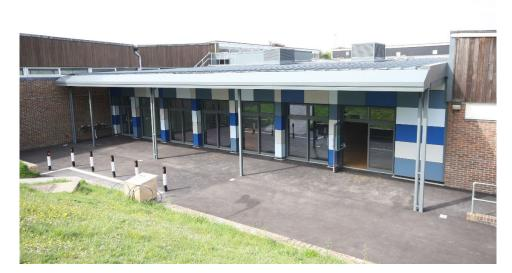
The project commenced on this restricted site with the RC ground bearing slab and the construction of a structural steel frame with an aluminium standing seam roof covering on metal profiled decking. The building façade is finished in insulated Rockpanel cladding.
