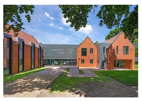
The first phase, comprising substructure and ground floor slab, carried out by the Sunninghill Groundworks and Civil Engineering Department, included the diversion of existing services, the installation of a new foul and storm water drainage system and piled and trench fill foundations. The second phase, the superstructure, comprised load bearing masonry and steel frame with curtain walling to the atrium; the roof a mixture of clay tiles and single ply membrane.
