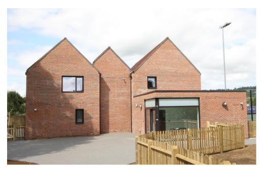
Construction comprised traditional concrete foundations, with a steel frame supporting the first floor, pitched timber roof rafters and structural metal walls. The external façade is brick, with large windows and sliding patio doors on the ground floor. Internal finishes include plasterboard walls and linoleum floor coverings with under floor heating.
