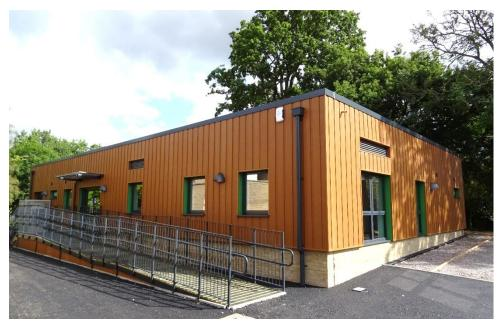
building was raised above ground and constructed on piled foundations due to its proximity to three large mature trees. The majority of the build was constructed within the root protection zone and the excavation works were overseen by an arboriculturist.
