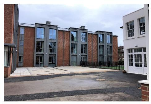
The building is steel frame construction with composite floor built up of precast concrete, insitu concrete topping and a floating timber deck floor to finish. The external envelope is formed in a steel frame system clad with a mixture of brickwork and zinc panels. The roof is pitched with loose fill timber rafters, insulated and completed with standing seam zinc panels including five ventilation towers.
