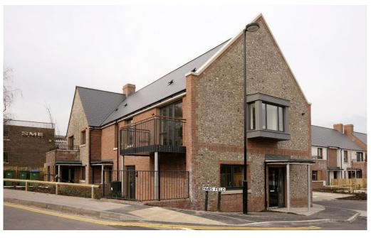
longer met today's standards. Work commenced with the demolition of the existing building, with material being crushed and reused in the new foundations. Of traditional construction the elevations are of brickwork and near white render, with knapped filed chalk flint blocks and timber reflecting the materials found in the nearby conservation area, but designed in a more contemporary style. The homes comply with the Housing Quality Indicator standards and with the principle of Lifetime Homes.
